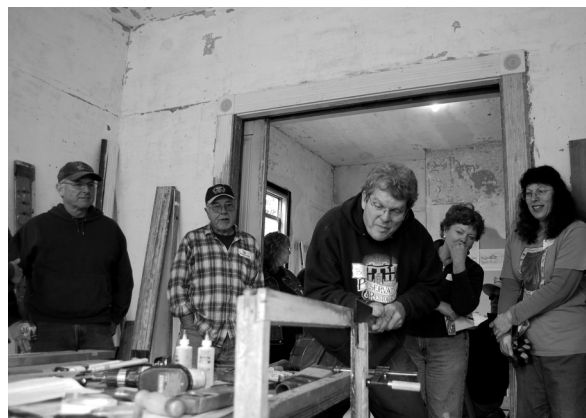
Mortise & tenon joint repair with Japanese saw
