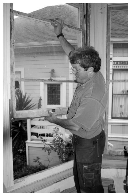
Bill Hole installs the repaired bottom sash.
