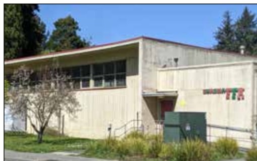
Eureka High School Ag and Welding building that cannot be saved. Heritage Society photo.
