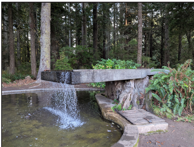
Usher's cantilevered concrete fountain in Sequoia Park.
